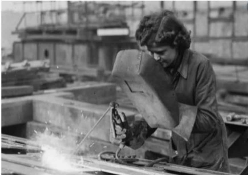
Female welders using elec-trodes, at Waterloo Bridge, London (UK) in 1944. Daily Herald Archive - National Museum of Science and Media - Science and Society Picture Library.
